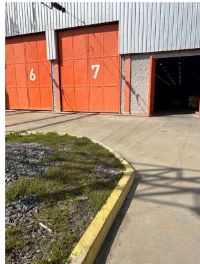
SECTOR DARSENA A DEMOLER
